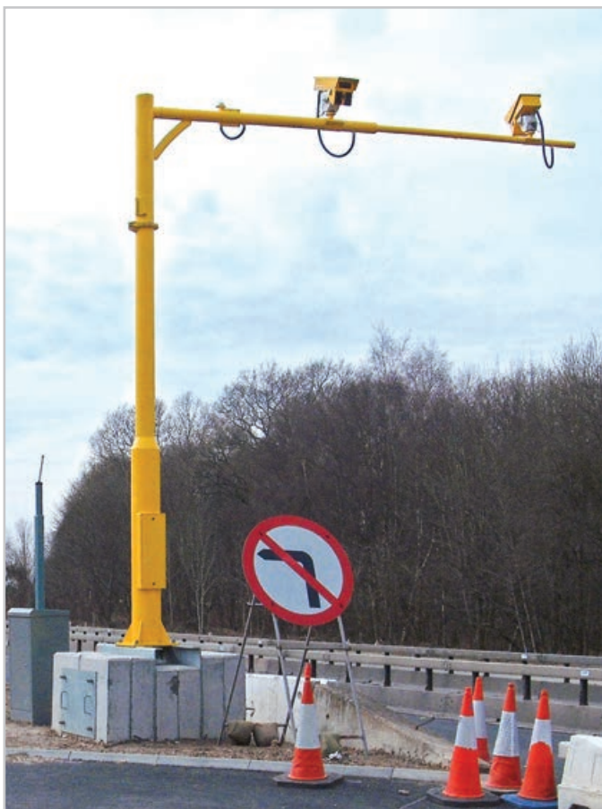
6m cantilever pole with 5m arm
