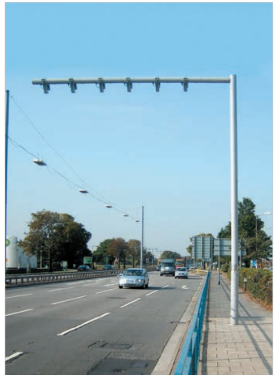
Low emission zone cantilever pole
