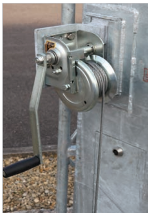
ANCT winch mounting arrangement
