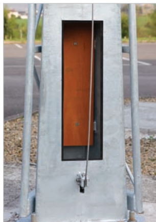
Large equipment mounting backboard
