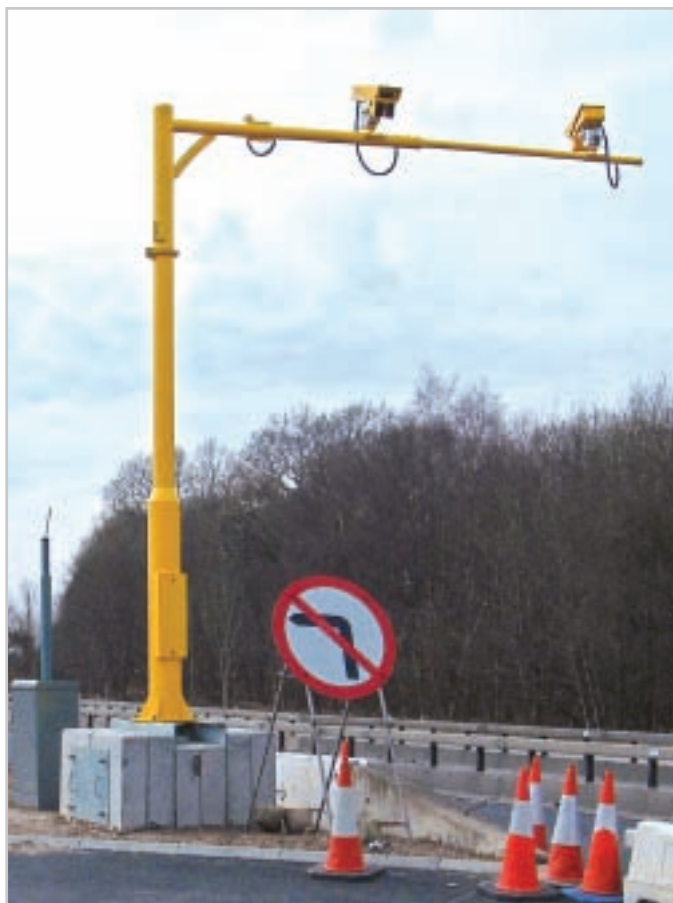
6m cantilever pole with 5m arm
